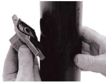
3. Gasket installation Insert the gasket into outlet housing properly. Align outlet housing over the pipe hole making sure that the locating collar is in the pipe hole.
