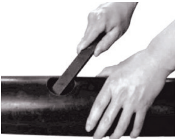
2. Remove burrs If any burrs or slug exists at the pipe hole, please remove them before assembly, to protect the gasket and avoid leakage.
