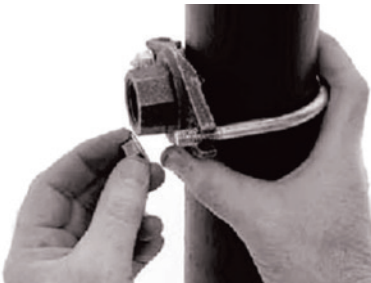
4. Alignment Attach the U-bolt from the other side and tighten the nuts finger tight.
